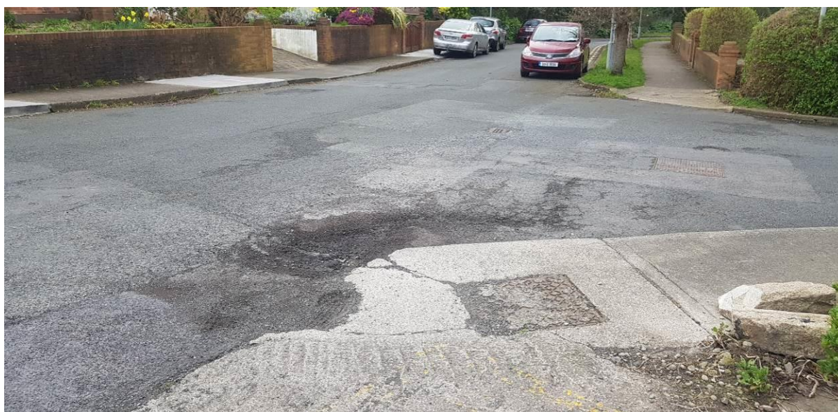
Figure 7: Poor existing surfacing at scheme tie-in
