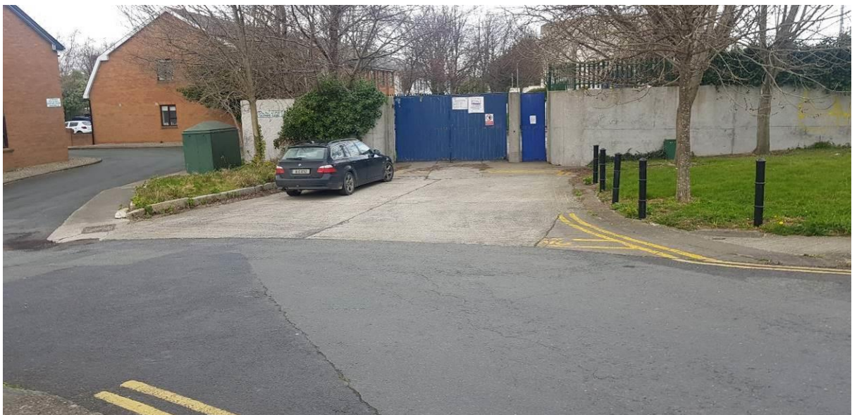
Figure 15: Existing Gate and Bollards at Pumphouse Access
