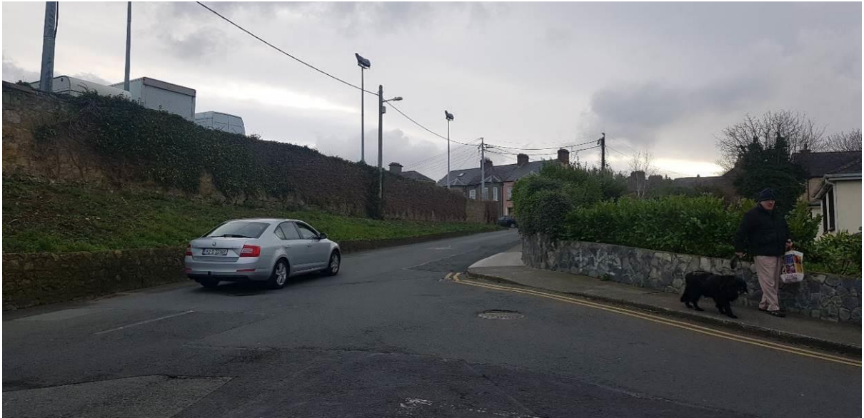
Figure 19: Poor visibility to right at Junction 2
