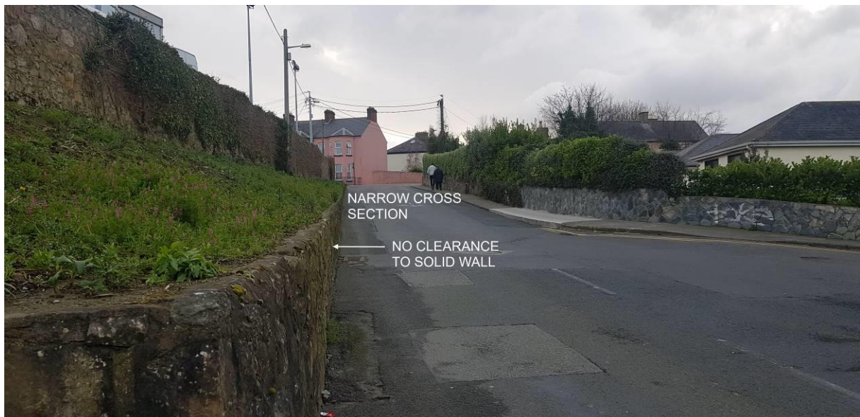
Figure 17: Narrow cross section with hazard immediately adjacent to carriageway
