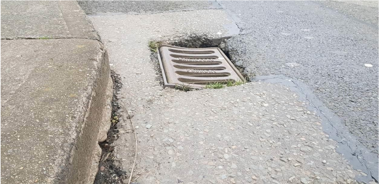
Figure 5: Sunken Gully at Location of Kerb Setback, Junction 2
