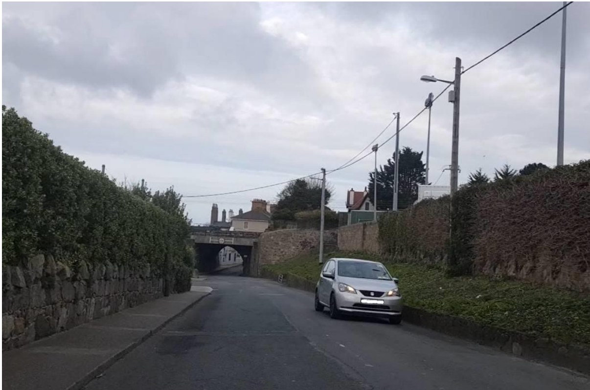
Figure 21: Current visibility on downhill approach to Junction 2
