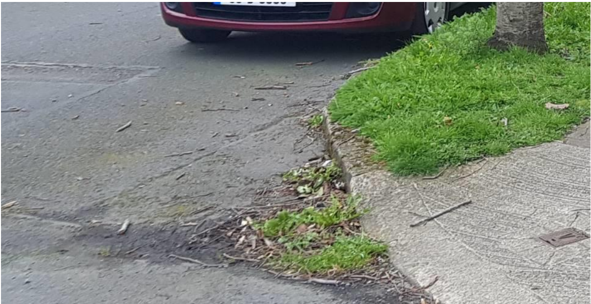
Figure 6: Blocked gully at scheme tie-in, Junction 2
