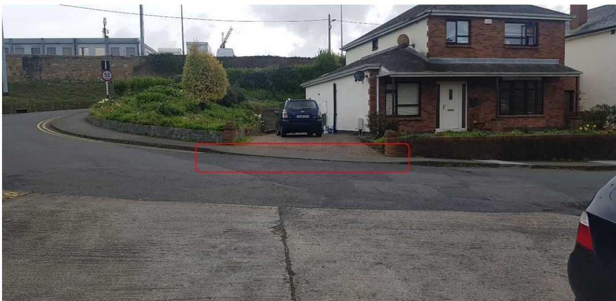
Figure 35: Existing dropped kerbs at private drive access
