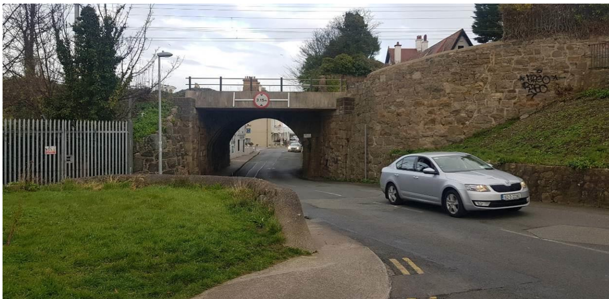
Figure 9: Dwarf Retaining Wall to be removed
