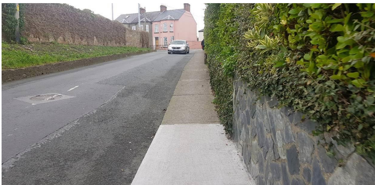
Figure 43: Existing footway narrow on cross section
