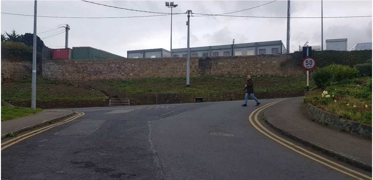
Figure 18: Rising levels and insufficient dwell area on approach to Seapoint Rd Junction
